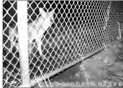
FIGURE 2. Coyotes are proficient at digging under airport fences that are not buried.
